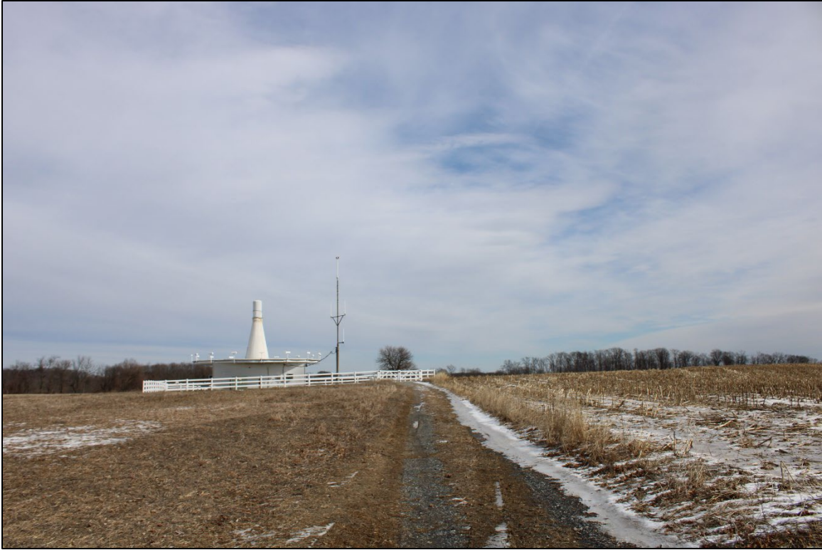
Photo 1. Looking northeast at the East Texas VOR/DME, located on cultivated farmland at the end of an unpaved driveway.
