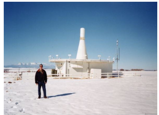
The author and the Dove Creek VORTAC (DVC) in southwest Colorado in February 2002.
