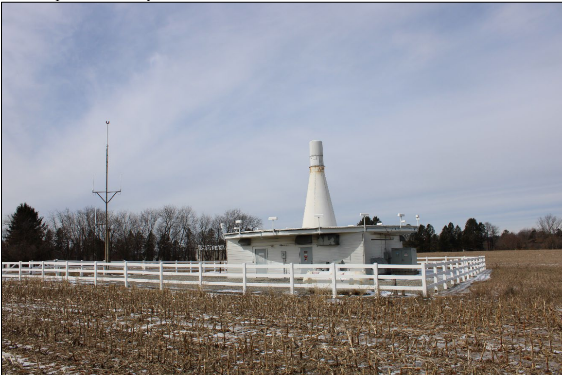
Photo 2. Looking northwest at the VOR/DME station, showing south and east elevations and the antenna at left.
